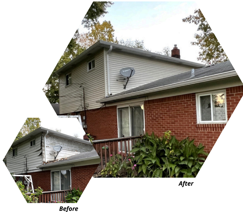
Siding Replacement, Project Sponsor: Federal Home Loan Bank of Indianapolis (FHLBI)
